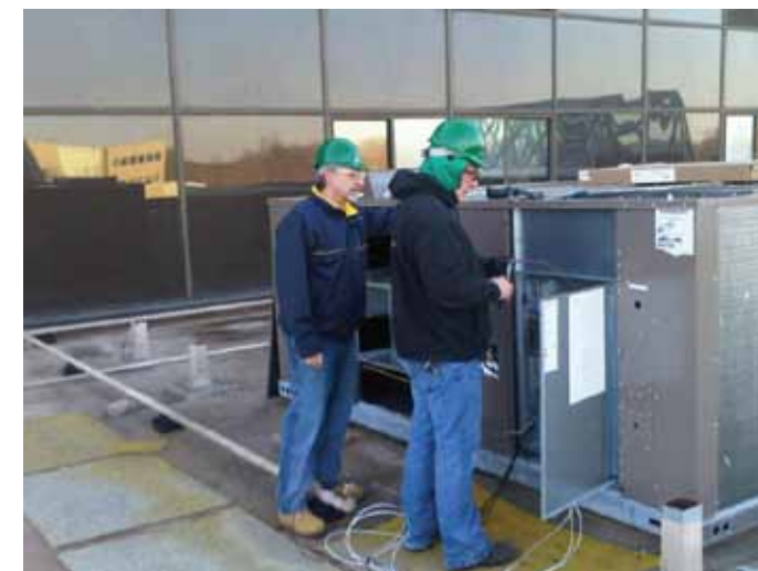
Service Installing a New Rooftop Unit at Virtua, Marlton, NJ Campus
