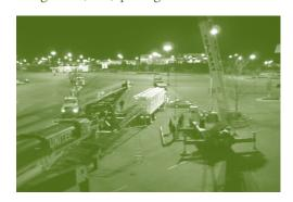
Chilled water rooftop air handlers were selected as the replacement. Utilizing the existing chilled water loop for the new cooling units will substantially reduce the electrical usage for this wing of the Mall.
